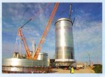
Ellimetal has built the largest aluminium silos ever in Europe with a capacity of 5000 m<sup>3</sup>
